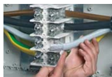
Conductor ends need to be rubbed with an acid and alkali free grease
