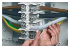
Conductor ends need to be rubbed with an acid and alkali free grease
